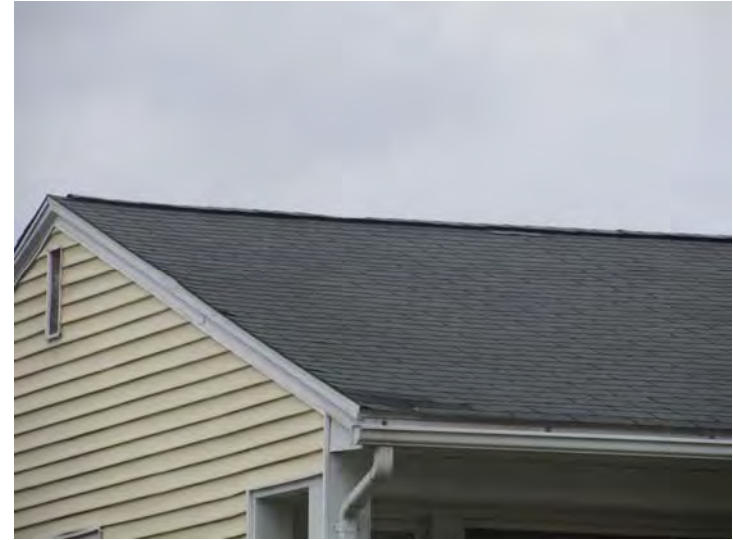
Roof shingles exhibit age-related wear/damage
