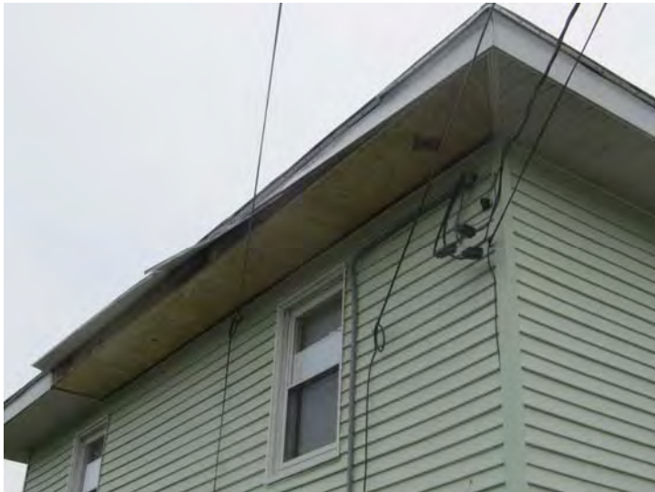
Areas of soffit damage noted at some buildings
