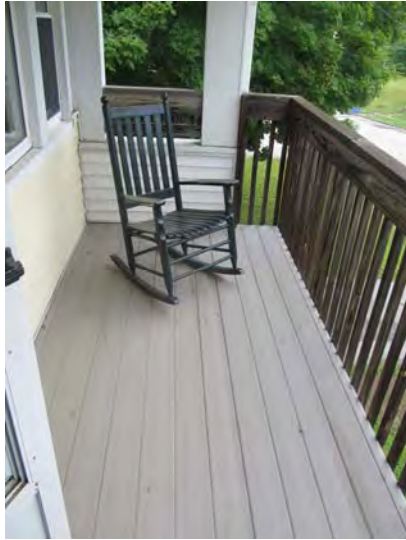
Newer, composite-type, decking typical on balcony surfaces at three-bedroom townhouse-style units
