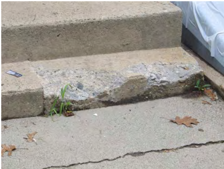
Concrete steps/stoops at unit entries are in need of repair at various locations
