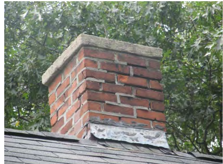
Worn/damaged chimney brickwork noted at several locations
