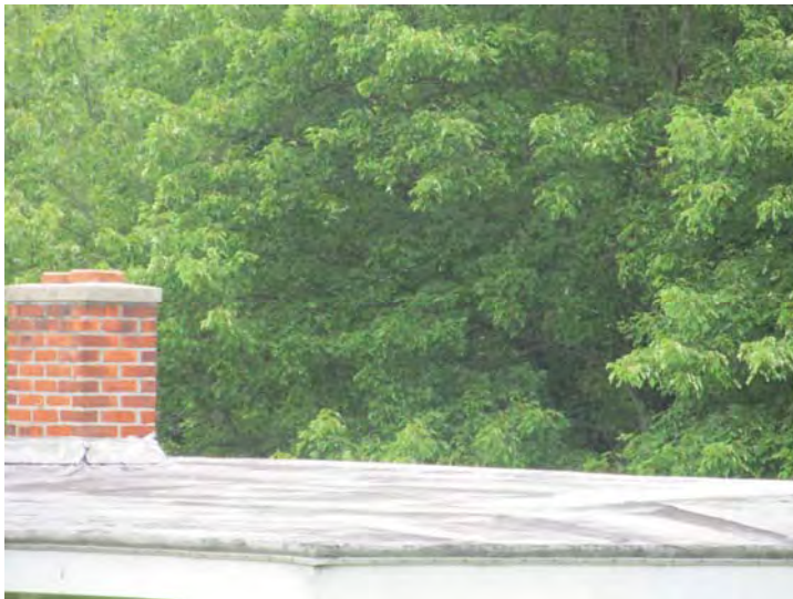
Coverings on flat roof surfaces also in need of replacement
