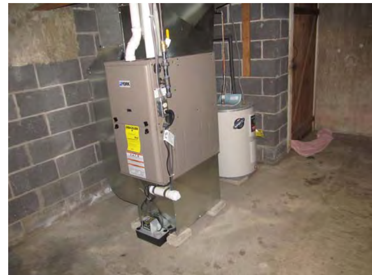
Typical warm air furnace and domestic hot water tank found at each unit – New furnaces recently installed in all units as part of conversion from oil to natural gas
